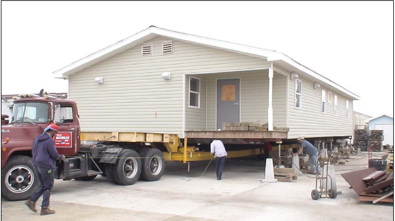
Workers from contractor Nick Martinolich, Inc. raise the building onto a trailer for transport down Veterans Blvd. to the permanent location at the Animal Shelter site.
